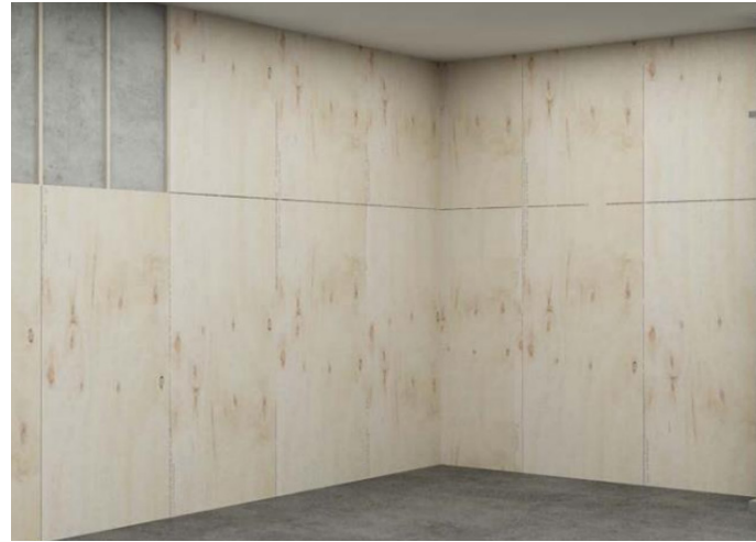
2. 9T PLYWOOD CONSTRUCTION
