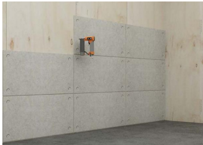
3. CONSTRUCTION OF STENCIL STAPLE GUN AFTER POSTON BOARD BACK WOODWORK BONDING WORK
