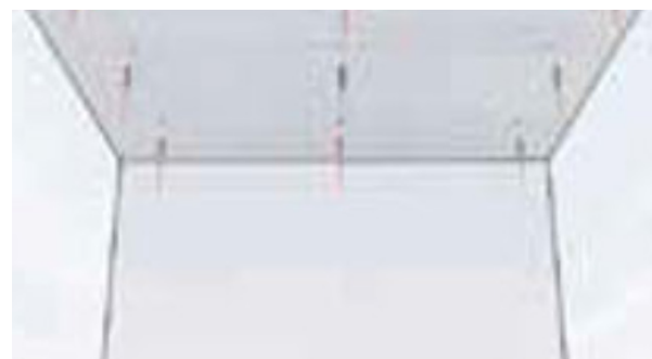
1. CENTERLINE ESTABLISHMENT AND ANCHOR CONSTRUCTION
