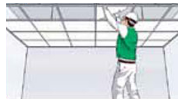
7. CONSTRUCTION OF FLAMEPROOF BOARD CEILING MATERIAL
