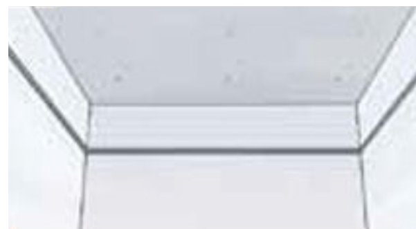
2. FRAME MOLDING CONSTRUCTION
