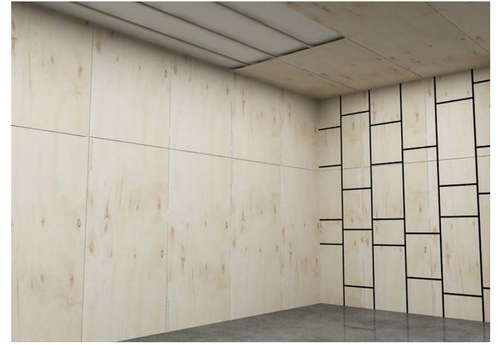
2. 9T PLYWOOD CONSTRUCTION
